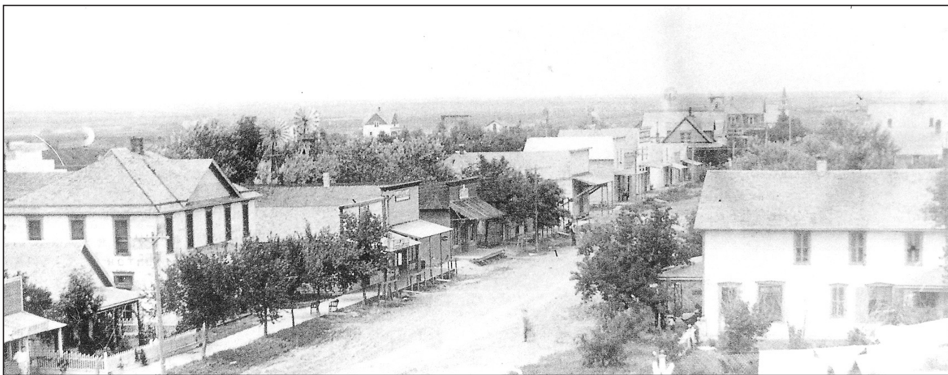
A BIRD'S-EYE VIEW of Dresden probably was taken from the top of the East Elevator. On the left, looking north: McIntyre Meat Market, Joseph Boeger home, the Caswell Hotel (later Bainter Hotel), Rhodes and Boardman Store, Still Brothers building, the Steel building, Muirhead Bank on corner,
