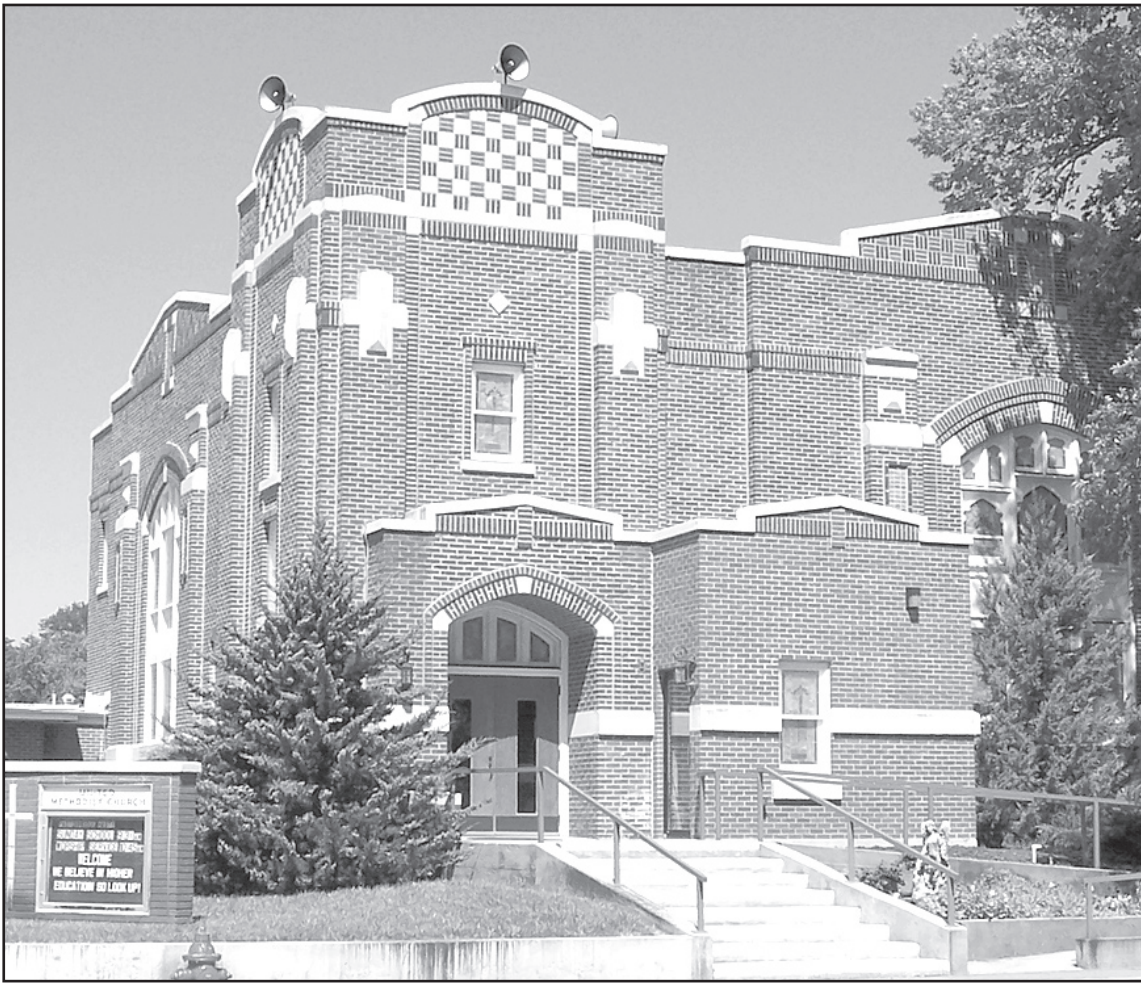
THE OBERLIN UNITED METHODIST CHURCH , above, was dedicated in 1926. Later an educational building was added. The congregation will celebrate the 130th anniversary of the church during morning worship services at 10:45 a.m. Sunday. — Church file photo
