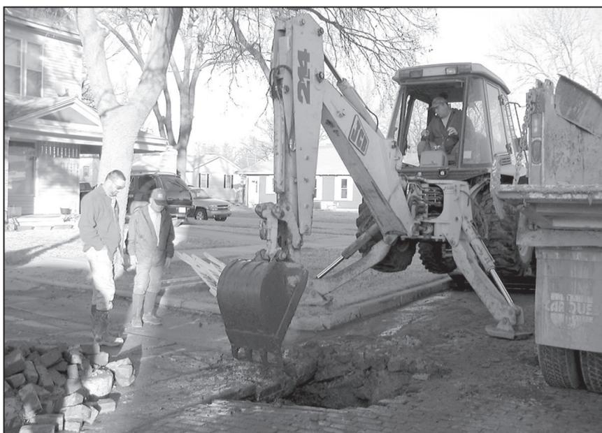
Norton City employees have been busy this fall fixing water leaks around town. Several of them are due to the extremely dry ground settling and causing strain on the pipes, causing the pipes to crack. This water leak on East Lincoln was caused by a bad spot in the pipe. City workers, Ed Lively and Cory Urban, watch as Steve Reedy runs the back hoe to clear the concrete. This must first be done so that the city crew can get down to the pipe in order to fix it.
