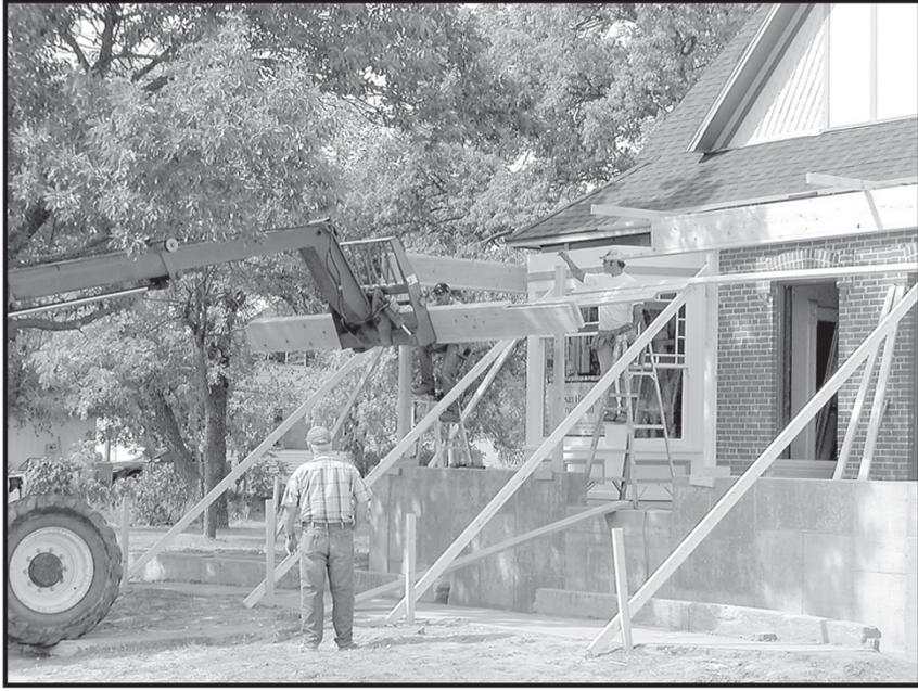
Schamber Restoration started work on the porch of the Lyons house this week. Lynn Schamber helps guide the lift operator in placing the front portion of the new porch as Brian Luther and Dave Turnbull position and attach it.
