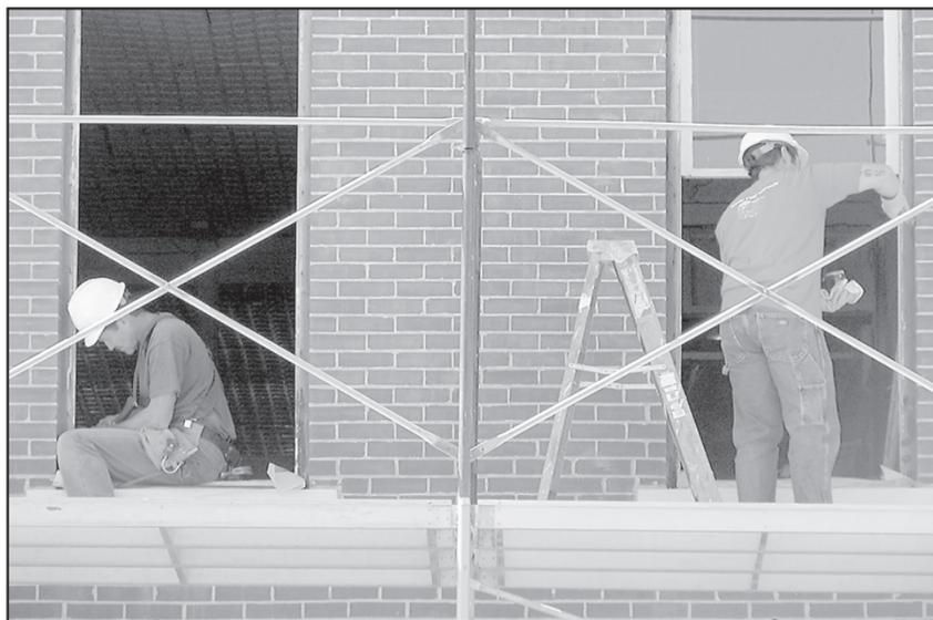
Renovation is in full swing at the downtown Heaton Building. Schamber Construction is renovating the building as part of the Norton County Community Foundation's renovation of the building, including the initial phase of tuckpointing, roof replacement, new soffatts, windows and doors.
