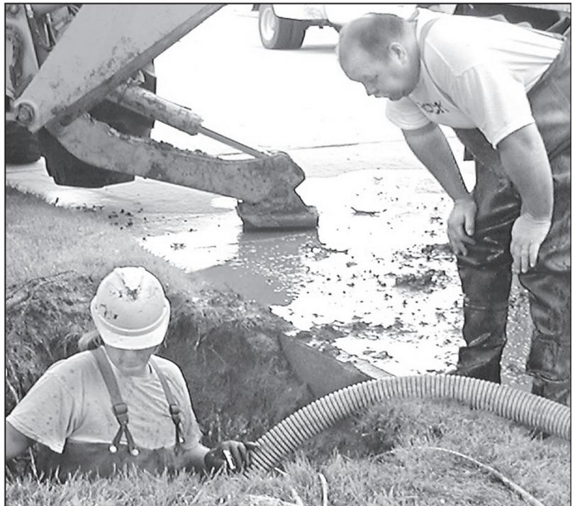
Jason Dial and Steve Reedy worked on fixing the water pipes on North Grant on Tuesday. The leak was fixed with a repair clamp after the crew evaluated the problem. Three water leaks were called in between late Tuesday afternoon and Tuesday night. The leaks are connected with work being done on the city's water tower.
