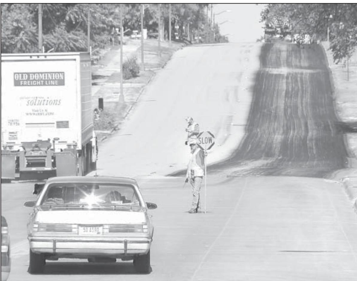
Traffic was detoured for awhile last Friday as Kansas Department of Transportation workers relaid a layer of asphalt on parts of U.S. 36 and U.S. 283. On U.S. 283 (above) traffic was reduced to one lane while other lane was overlaid with asphalt and sand (right).
