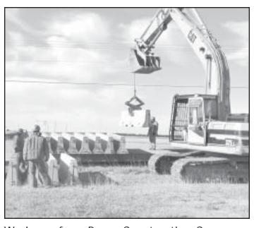
Workmen from Reece Construction Company, Scandia, removed the cement barrier walls from the bridge construction project on the west edge of Norton. Here, they unload the 4,000 pound barriers and stack them on a side lot, waiting to be used again in the spring when the next bridge, west of
