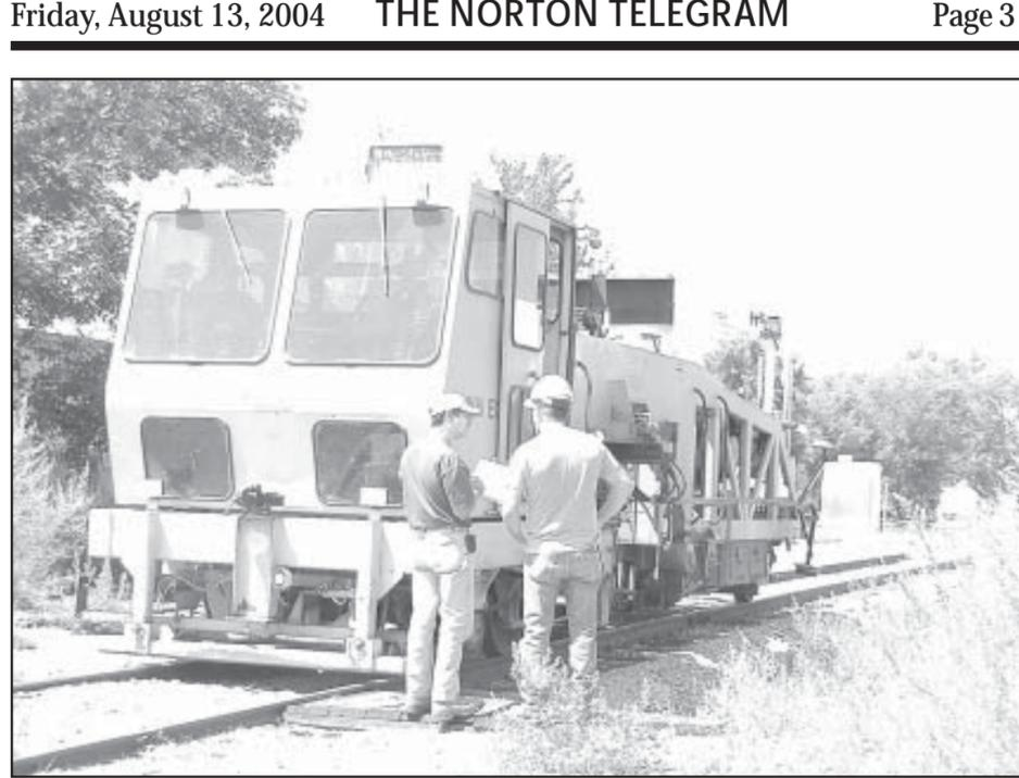
Monsters roared down the rails in Norton on Thursday as track crews for the Kyle Railroad used a "tamper" (right) to lift rails and ties and a "ballast regulator" (above) to straighten the alignment of the tracks, fill in holes and reshape the ballast. The machines can fix one and one-half mile of track a day. — Staff photos by Cynthia Haynes
