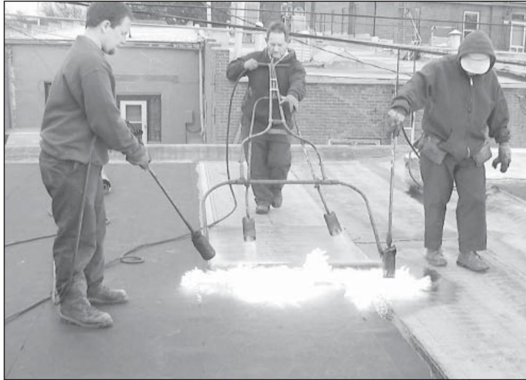
Workmen from Knoll and Sons Roofing Co. used propane torches to heat the back of new roofing material they laid on the roof of the Carter Building, 213 S. Kansas last week. A company spokesman said they removed over 40,000 pounds of tar and rock from the old roof in preparation for the new. —Telegram photos by Carolyn Plotts
