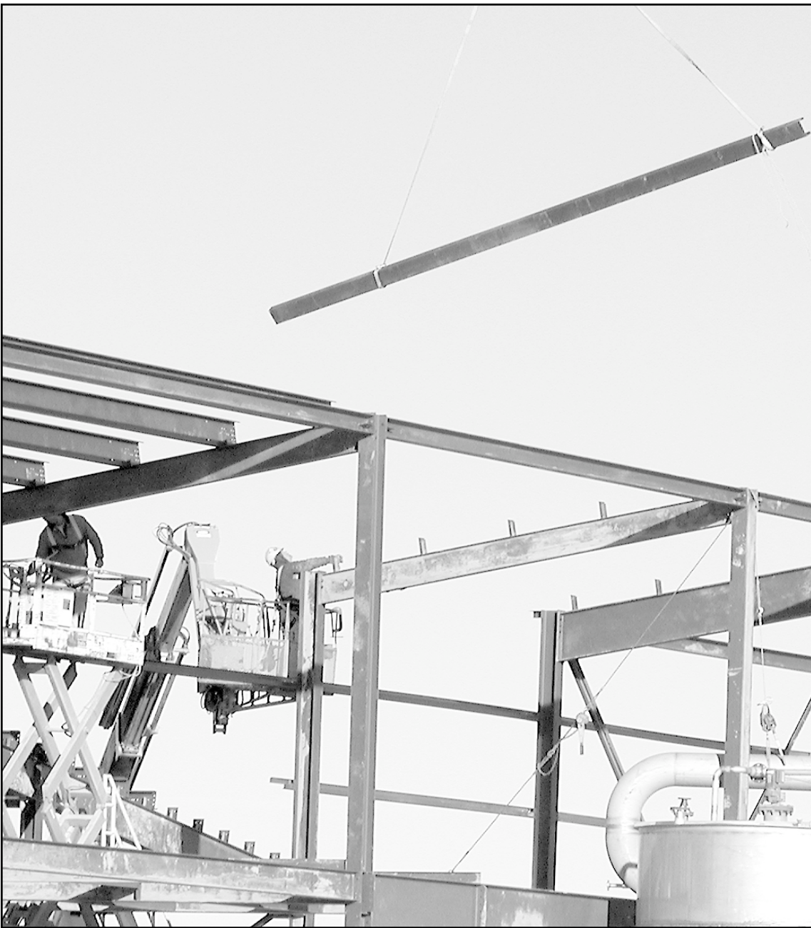
Steel sections are being lifted into place on the building at the ethanol plant at the Goodland Energy Center. Project Manager Roger Marsh of IMC Engineering told Goodland High School students that many of the tanks for the ethanol process are in place, and other are ready to be installed.
