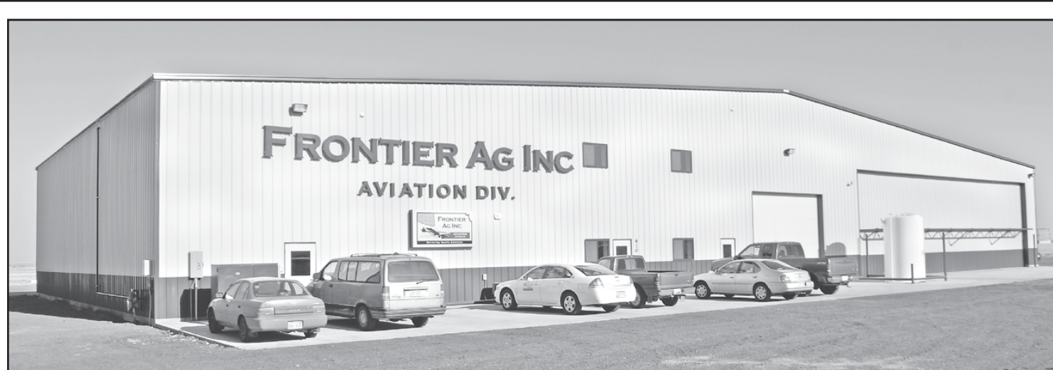
The new Frontier Ag hangar at the airport has space for planes, maintenance and chemical storage and loading all on the inside. The 17,000 square-foot structure is nearly complete. Photo by Kevin Bottrell/The Goodland Star-News
