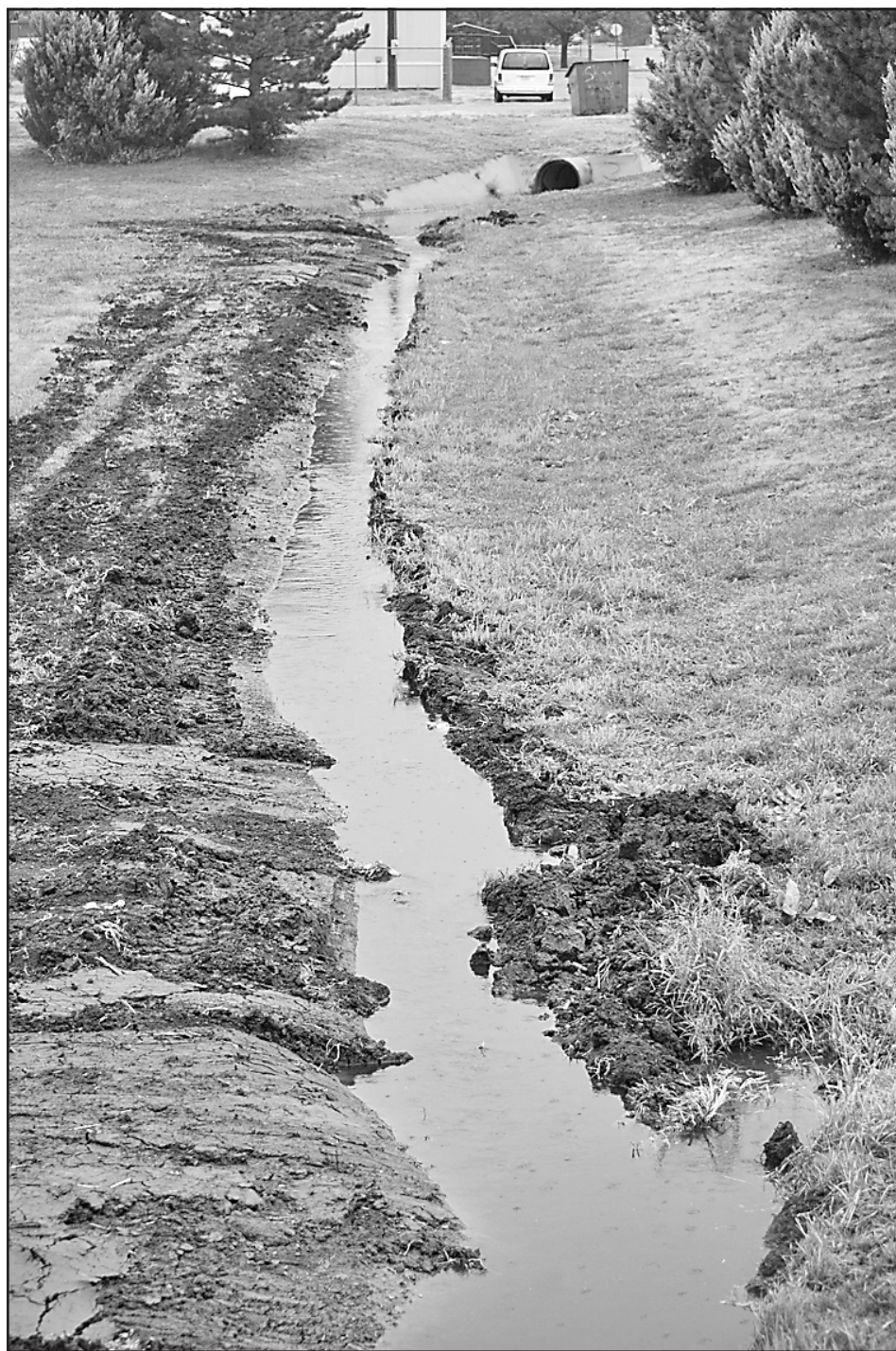
A lot of the water drained into this trench in the retaining pool by West Elementary School. This pool and others like it are designed to take water off the streets. Photo by Kevin Bottrell/The Goodland Star-News
