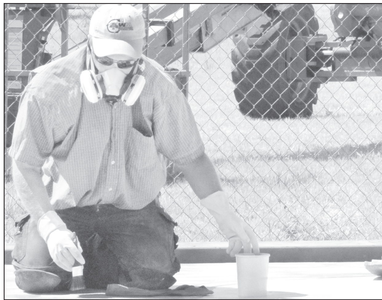
Under his purple awning, Cross mixed the chemicals he needed for his filler formula, which allowed him to paint over the screw holes and seams.
