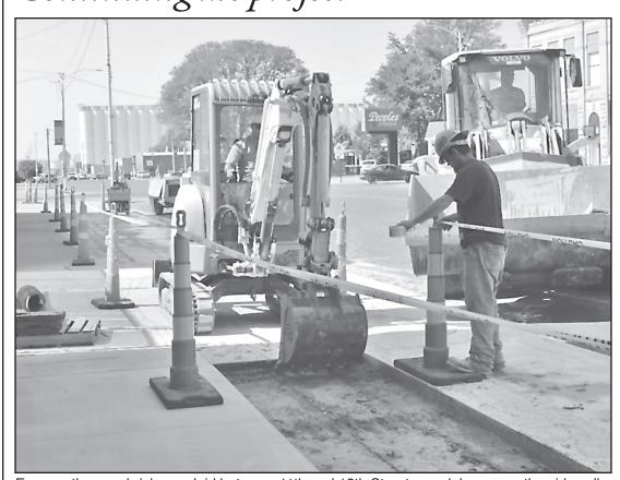
Even as the new bricks are laid between 11th and 12th Streets, work began on the sidewalks between 12th and 13th Streets. Crews have been tearing out part of the concrete in order to lay new water pipes under the sidewalk. Photo by Pat Schiefen/The Goodland Star-News
