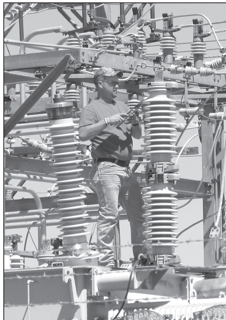
Taking apart the old transformer (above) to use parts on the replacement (top photo). The old transformer (right) after being moved.
