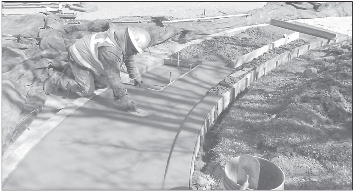
APAC of Hays crews continue working on the curb and gutter and valley gutters on Caldwell Ave. getting the street ready for the upcoming mill and asphalt overlay to be done this spring.
