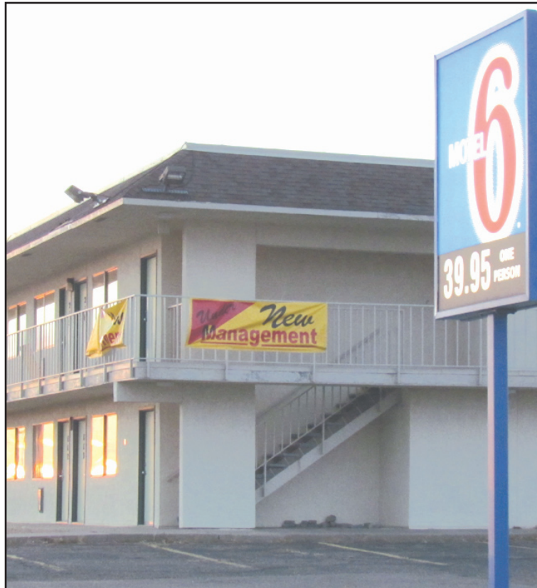
Lights are back on at Motel 6 on Commerce Road, and plans were presented to the city for more renovation and improvements.
