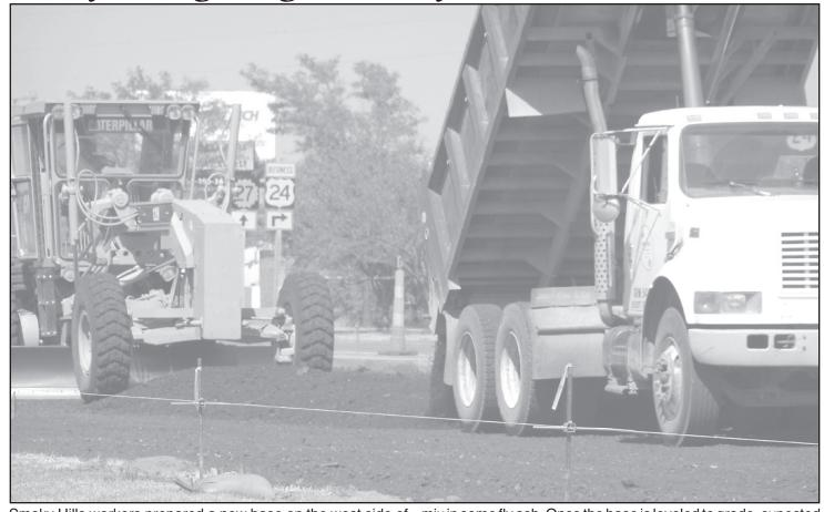
Smoky Hills workers prepared a new base on the west side of K-27 from the Walmart entrance to the north intersection. Smoky Hills put some asphalt milling down to be part of the base, and will add to the base to bring it up to grade and the next step will be to
