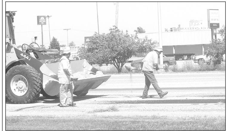
Maintenance workers for the Kansas Department of Transpor- the lanes. The section of highway from the intersection south to tation were throwing sand on top of new strips of asphalt on I-70 is slated to be replaced over the next few years through an Wednesday where the travel lanes had been milled off to smooth improvement program. Photo by Tom Betz/The Goodland Star-News
