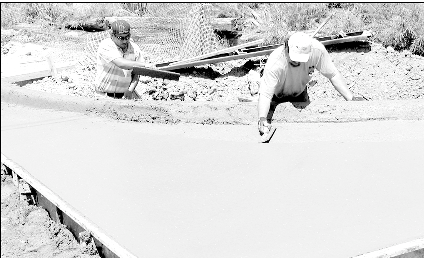
Workers for Spore Land Development smoothed the new curb on the east side of Broadway and 17th on Tuesday. The project is moving down the north side of 17th, and Jerry Nemecheck from Evans, Bierly, Hutchison and Associates inspecting the
