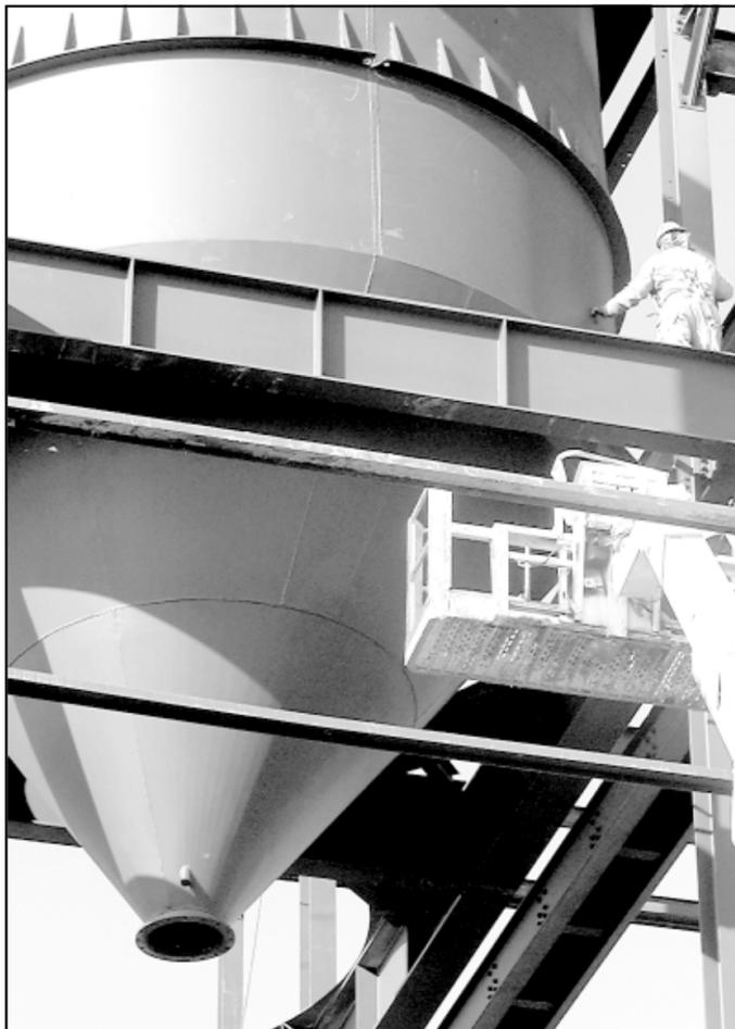
A steel worker (above) reached out to steady a coal bunker as a crane from Belger Cartage Service of Denver lowered the 32,000-pound piece of the power plant into the steel collar Wednesday afternoon. The 200-ton crane (right) lifted the coal bunker high into the air to get it into position. A second coal bunker was lifted into place Thursday morning. Photos by Tom Betz/The Goodland Star-News
