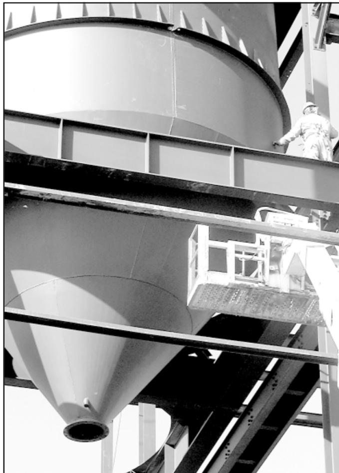
A steel worker (above) reached out to steady a coal bunker as a crane from Belger Cartage Service of Denver lowered the 32,000-pound piece of the power plant into the steel collar Wednesday afternoon. The 200-ton crane (right) lifted the coal bunker high into the air to get it into position. A second coal bunker was lifted into place Thursday morning.
