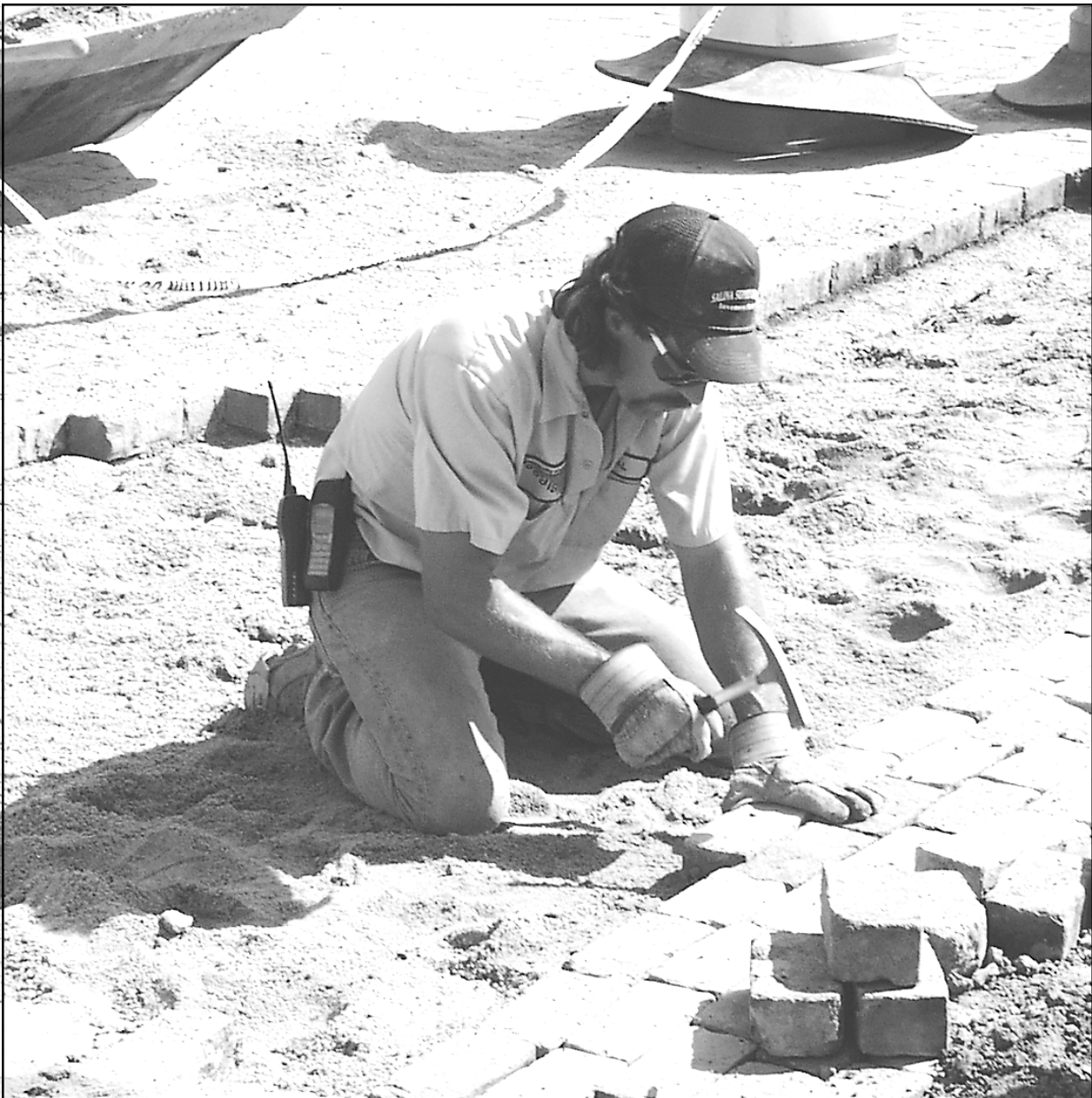
Neil Thornburg, with the Public Works department, hammered bricks back into place after the crew repaired a pipe under Main street. Photo by Reaghan Smith/The Goodland Daily News
