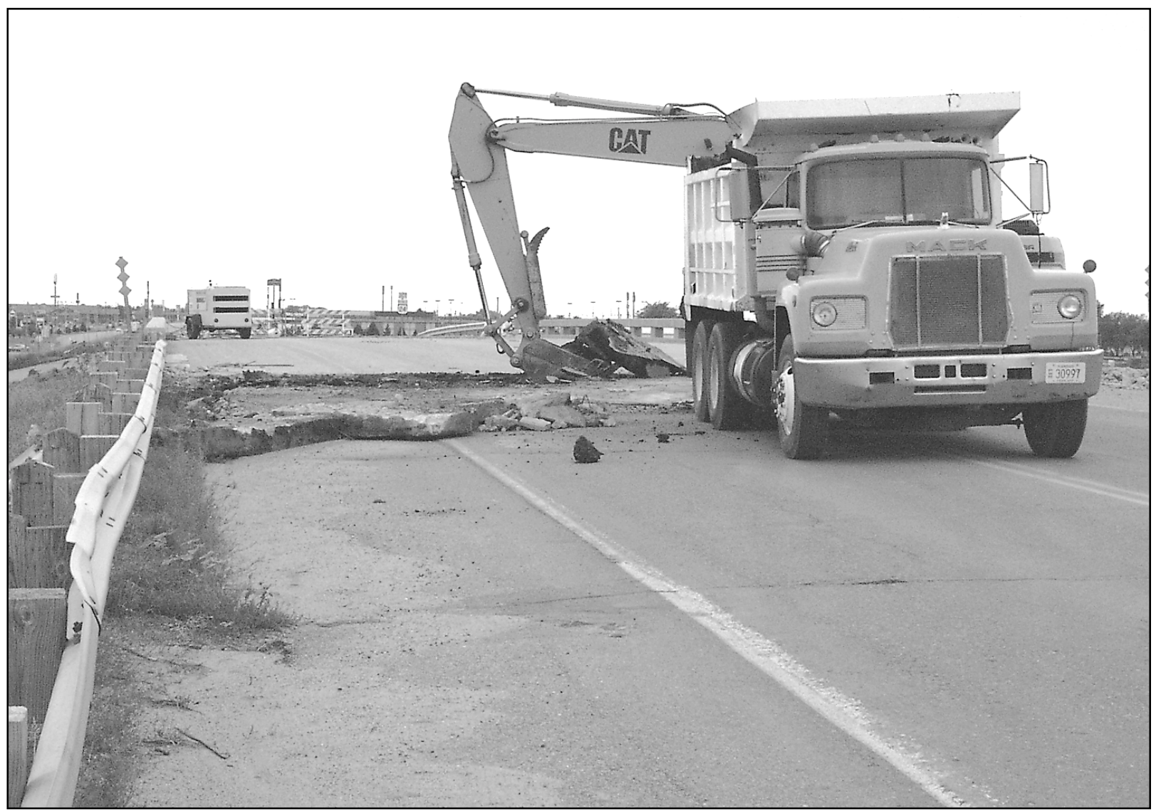
Construction progressed on the railroad viaduct on K-27 today with asphalt being lifted to make room for the new approach slabs. The construction coinciding with the Cherry Street project has caused traf-
