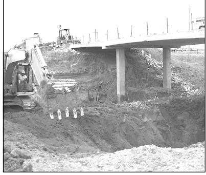
Concrete guardrails have already been removed from the first bridge north of Goodland, which will be widened.
