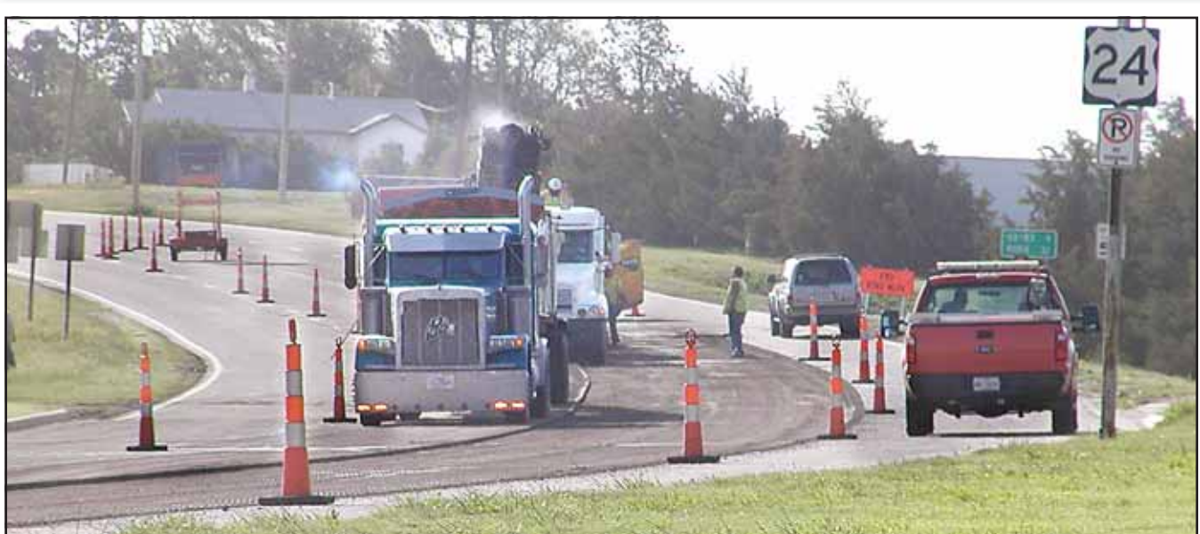
SAM DIETER/Colby Free Press Road crews from McCormick Excavation and Paving started milling off the asphalt in the middle of Fourth Street Tuesday morning (below), and finished laying down new asphalt in the middle of the street that afternoon, starting on the north lanes Wednesday. By Thursday morning, they had moved onto east Fourth, out to the city limits (above), and they plan to finish work on south Range, the last part of their project, next week.
