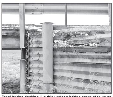
Steel bridge decking like this under a bridge south of town on K-25 is rusting out, forcing the state to replace it this spring. The span will be closed during harvest, but should reopen
