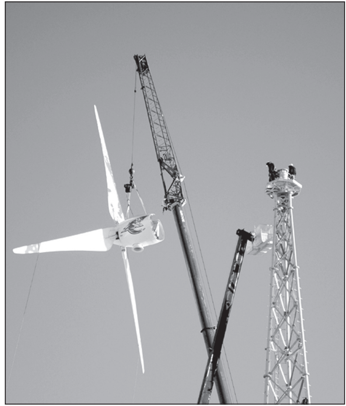
LYNN CAMERON/Colby Community College Woofter Construction crew members stood on top of the 140-foot tower last week preparing to install the 50-kilowatt wind turbine on the east side of the Colby Community College campus. Each blade is about 30 feet long. The turbine will provide electricity to Living Center Northeast; it is part of a $4.5 million project to reduce energy consumption. The turbine is projected to produce 193,000 kilowatt-hours in the next 12 months – about 54 percent of the needs at the residence hall. In addition, the project will provide internship opportunities for students.
