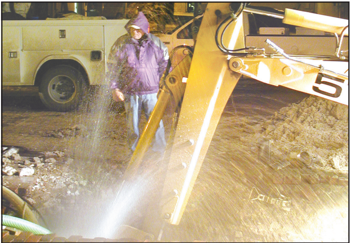
EVAN BARNUM/Colby Free Press Crews worked late into the night with a back hoe, jackhammers and pumps, trying to repair the break. A large hole had to be dug in Fifth Street to get at the water main.
