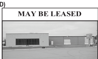
1675 W. 4th 6,000' office + 4,500' warehouse Give Pat a call today!!!
