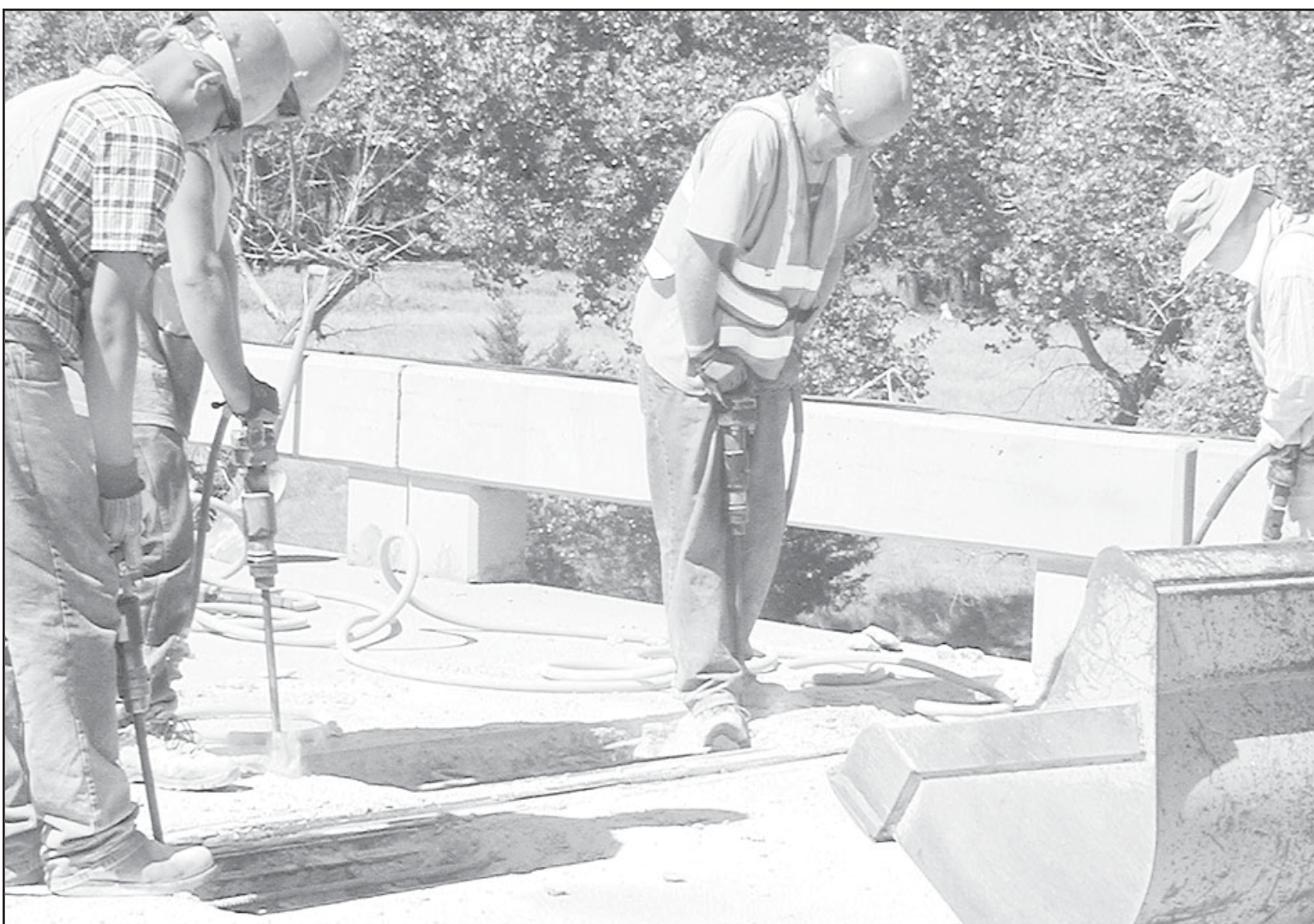
WORKMEN BEGAN JACKHAMMERING the concrete around the joints of the bridge west of St. Francis on Tuesday. Travelers were slowed down when they wait for the stop light as only one-lane traffic is allowed. Herald staff photo by Karen Krien
