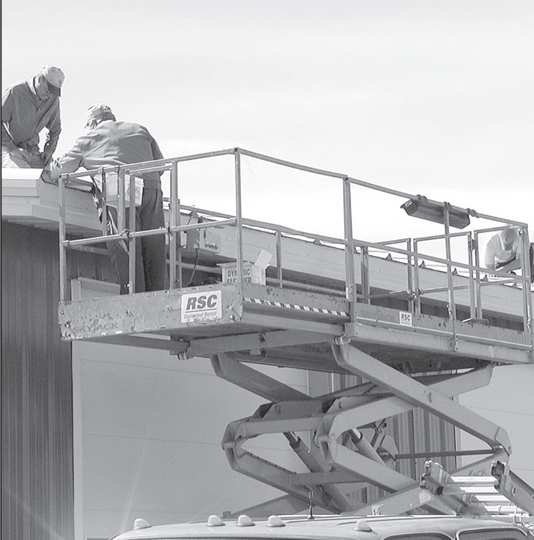
SNOW GUARDS AND GUTTERS are being installed on the St. Francis Emergency Building on U.S. 36. The ice built up from snow dripping on the roof onto the north side of the building has been a problem. Krien Steel Building crew, left to right, Dale Carpenter, Ron Krien and Sam Reed are doing the work. Herald staff photo by Tim Burr
