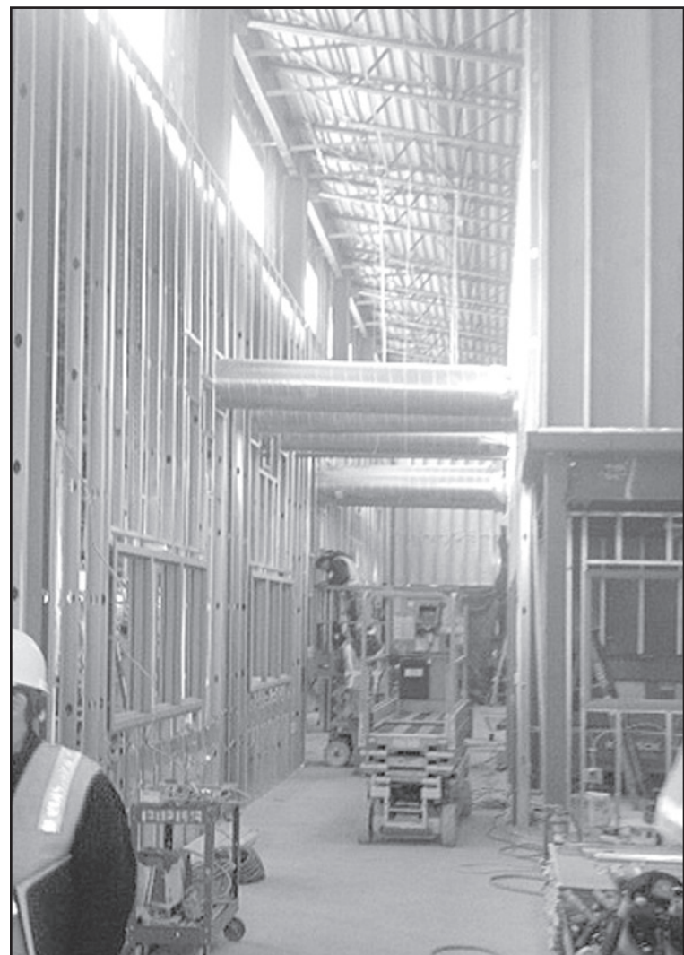
CONSTRUCTION is moving along at the Idalia school.
