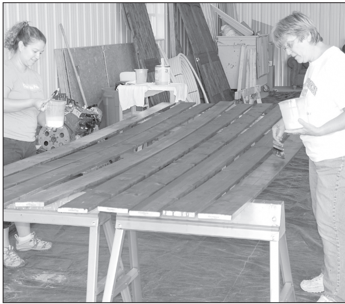
VOLUNTEERS – Jess Andrews, left, and Deb Crites seal the baseboards for "The Grainery," the new restaurant being built in Idalia. The restaurant is scheduled to open in August. Crews of community volunteers will continue to work daily to complete the baseboard project by July 24.
