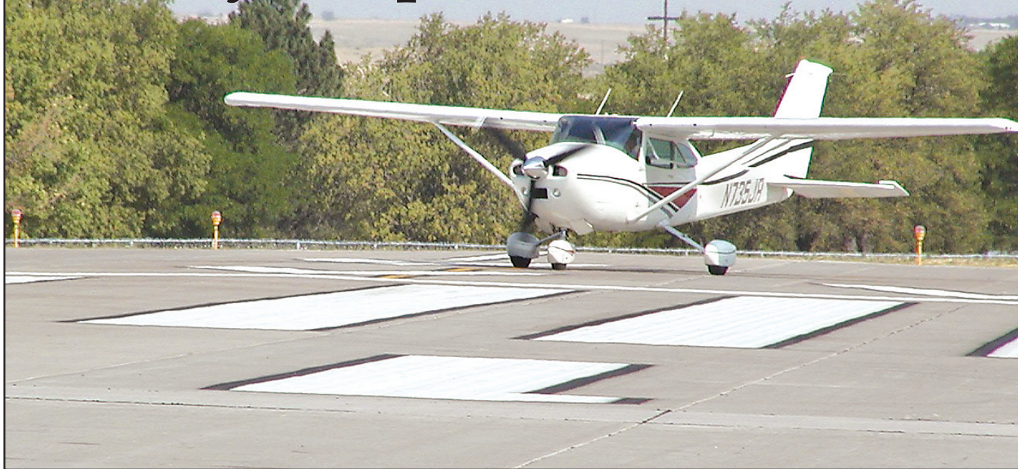
CHEYENNE COUNTY RUNWAY is officially open for business. The new runway, constructed of concrete, is longer and wider, and able to handle the air traffic coming into the county. Look for more information next week.
