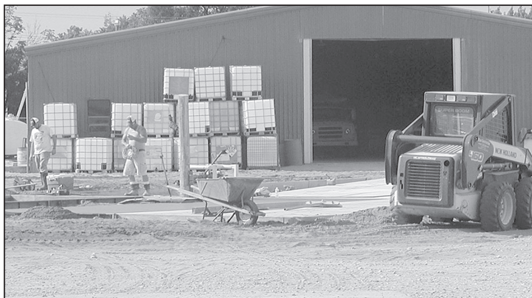
THE ST. FRANCIS EQUITY is putting in a chemical loading pad.
