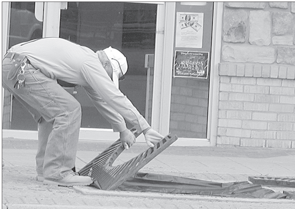
ERIC FIALA, city employee, removes the grate and fills the empty tree hole with pea gravel. Herald staff photo by Karen Krien
