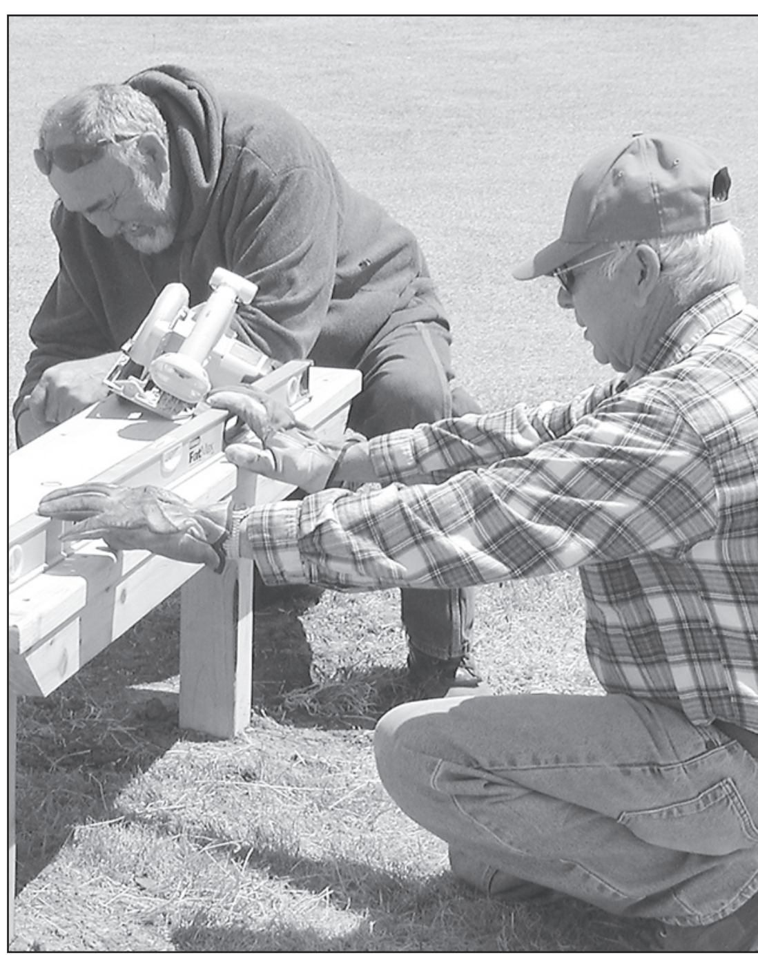
Rod Klepper donated the time and materials to build new benches for the Bird City Golf Course. Ray (left) and Willy Martinez (right) volunteered their time to build them. They are done and really spruce up the golf courses just in time for the Golf Tournament to be held at the Bird City Golf Course on May 21.
