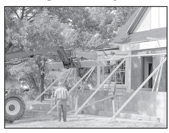
Schamber Restoration started work on the porch of the Lyons house this week. Lynn Schamber helps guide the lift operator in placing the front portion of the new porch as Brian Luther and Dave Turnbull position and attach it.
