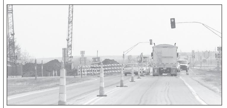
Work is in full swing on Highway 36 east of Norton where Kansas Department of Transportation crews are working to overlay about four miles of roadway. The bridge east of town is down to one-lane traffic and controlled with a stoplight. Drivers are urged to use caution in the construction zone and be aware of workers in the area. -Telegram photo by Dana Paxton
