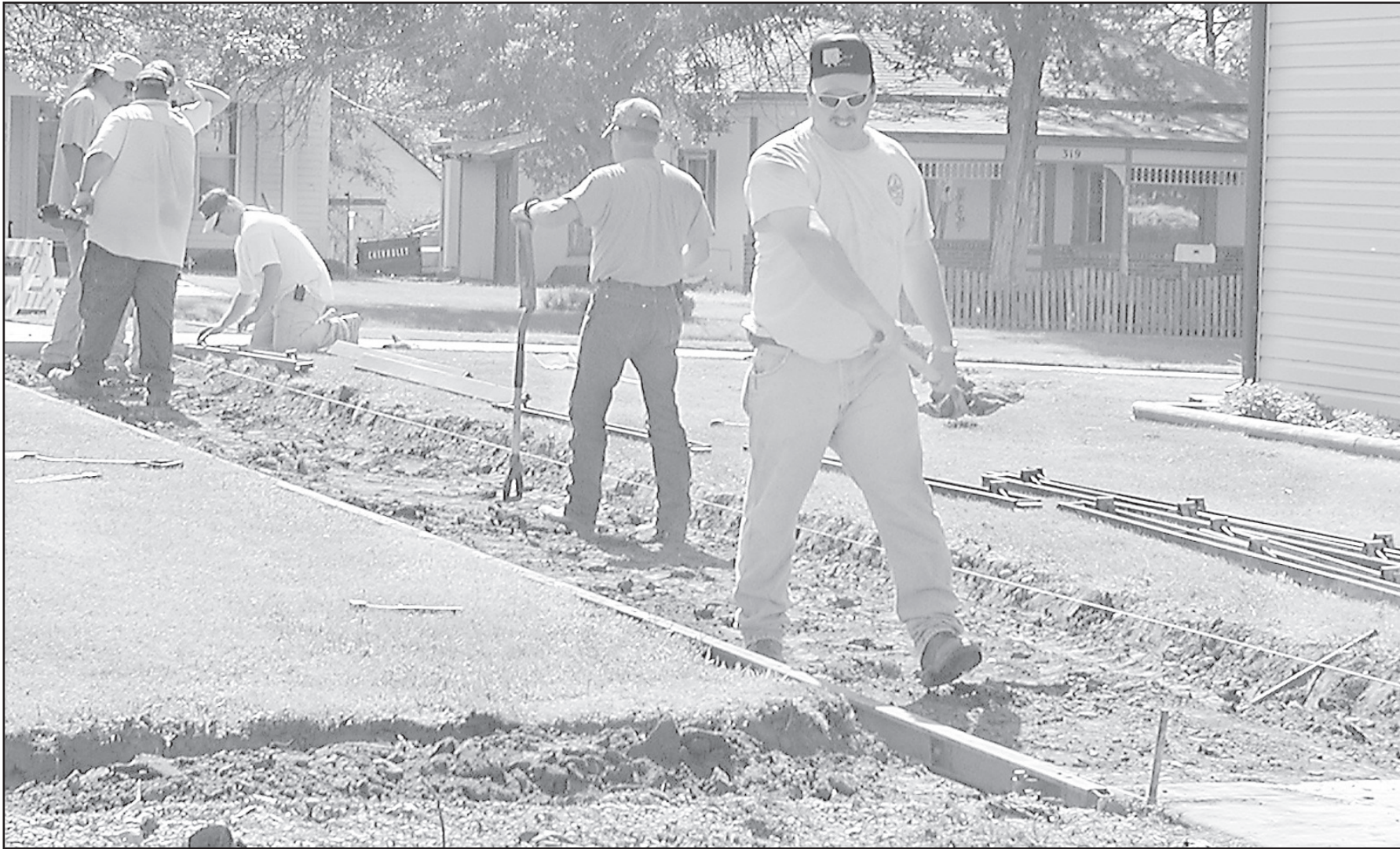
City crews worked on pouring concrete at Jeff Wolf's residence last week. Crews frequently work on sidewalk replacement throughout
