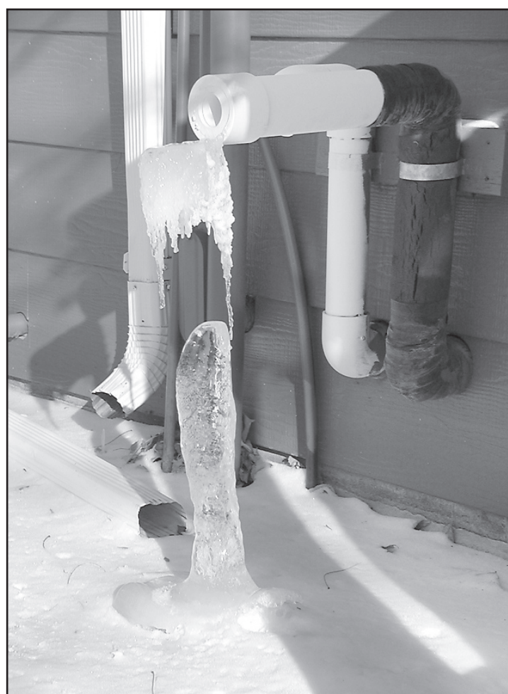
Temperatures fell across the country this week with many homes being affected when even steam from dryer vents froze. Temperatures remained below freezing all week but were expected to climb into the 40's early next week.
