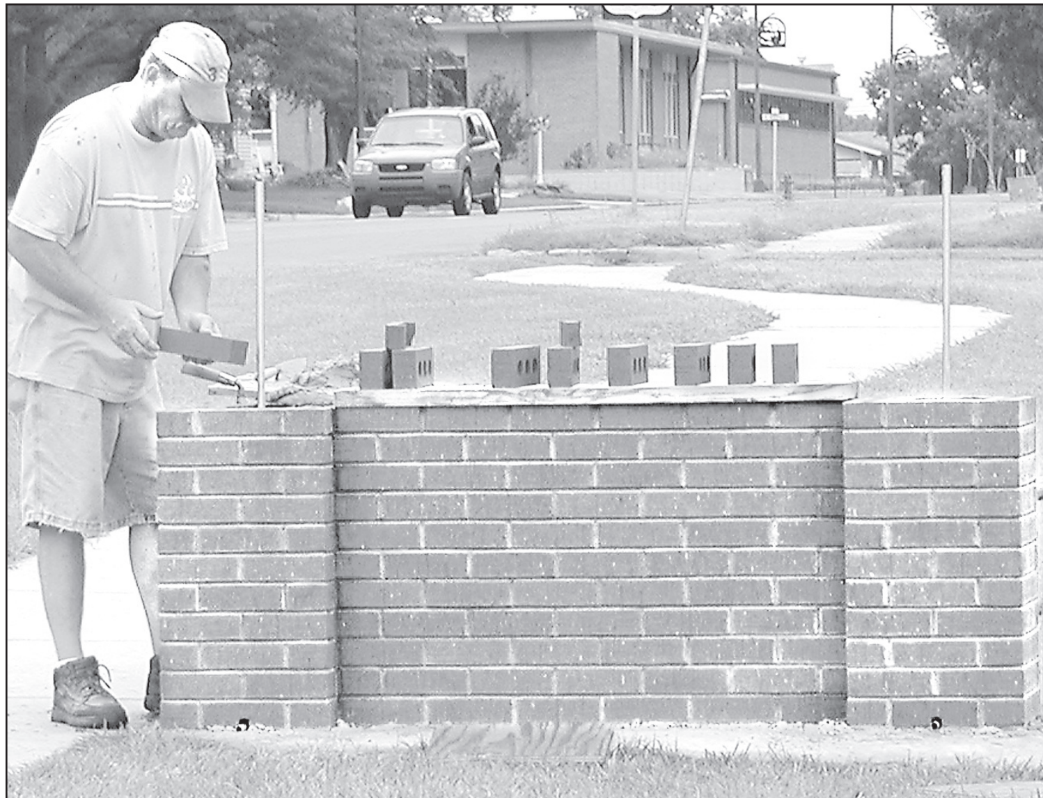
Jeff Jones placed brick for the new sign in front of the Norton "Norton Library." Public Library. There will be six-inch lettering proclaiming
