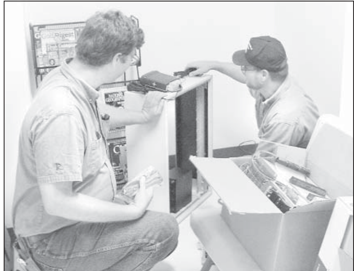
Kevin Strutt (left) and Vance Scott with Nex-Tech's mobile radio department installed a new base station at Norton County Hospital Tuesday. The base station, a new remote and a repeater on a tower south of town, are all part of the hospital's new paging system that it got with a bio-terrorism grant this year. The new system will make it possible for emergency personnel to contact the hospital from almost anywhere in the county.
