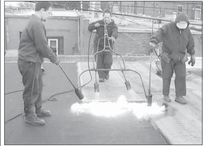
Workmen from Knoll and Sons Roofing Co. used spokesman said they removed over 40,000 propane torches to heat the back of new roof- pounds of tar and rock from the old roof in prepaing material they laid on the roof of the Carter ration for the new. Building, 213 S. Kansas last week. A company
