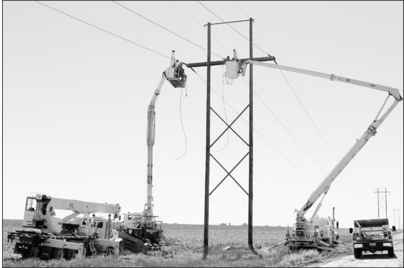
SUNFLOWER ELECTRIC POWER SERVICE crews were working to repair the transmission line that was knocked down in the strong wind storm.
