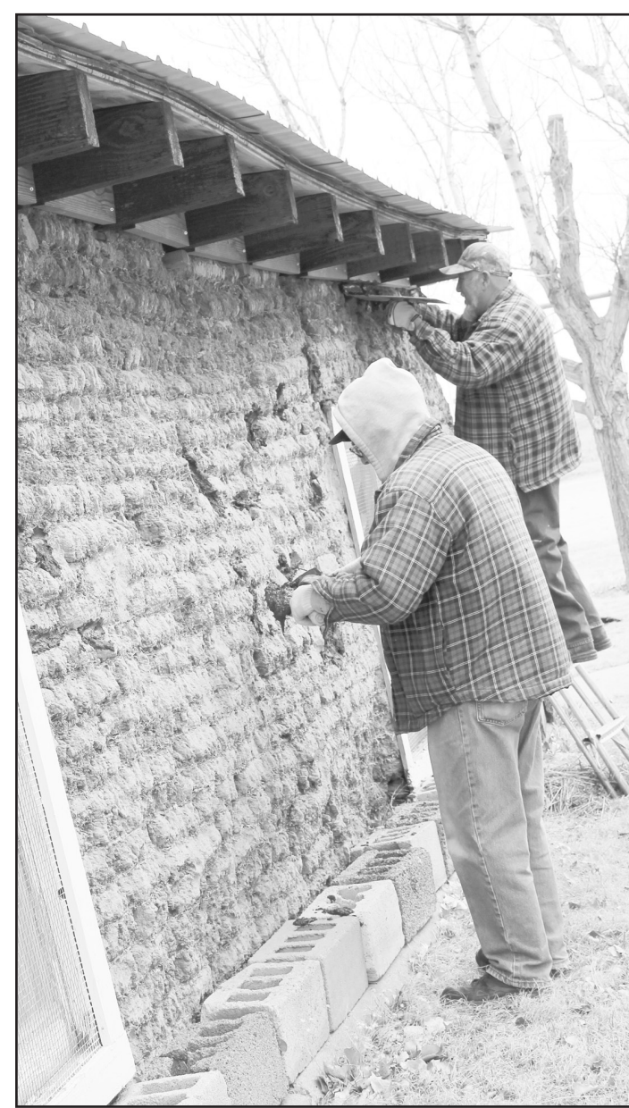
LAST SATURDAY Willy and Ray Martinez were seen at the Thresher show grounds dressed in winter clothes, mixing mud and filling in the holes in the sod house. As soon as the winds die down and the temperatures are more stable, the grounds will be full of workers constructing the new building and cleaning in preparation for the July 4 celebration, and the thresher show events.
