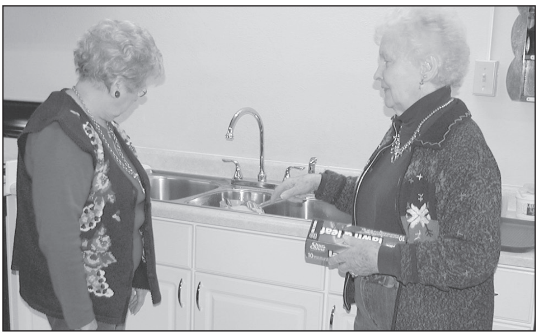
DEE DORSCH is showing Edna Roesener the garbage disposal in the new sink recently installed in the Senior Center.
