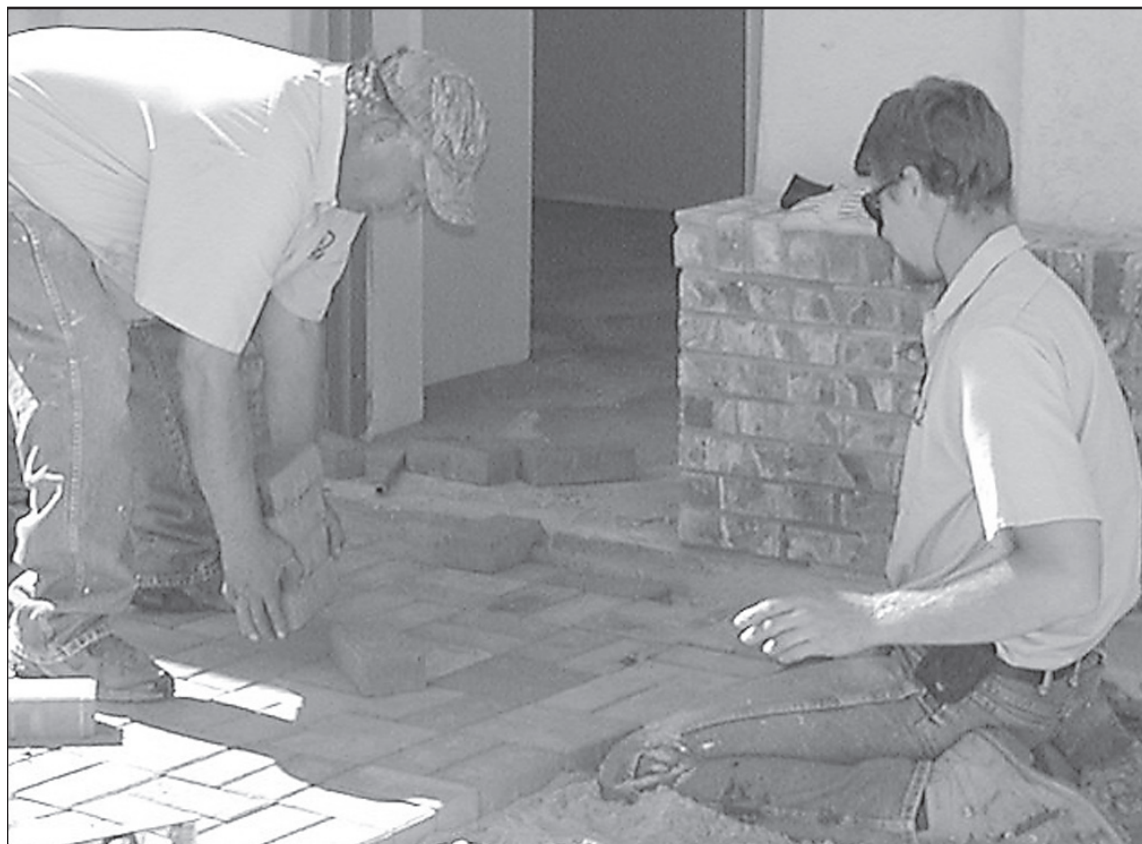
BRAD SCHNEIDER and Russell Jackson are filling in the holes at the Legion hall with brick as a temporary fill in.
