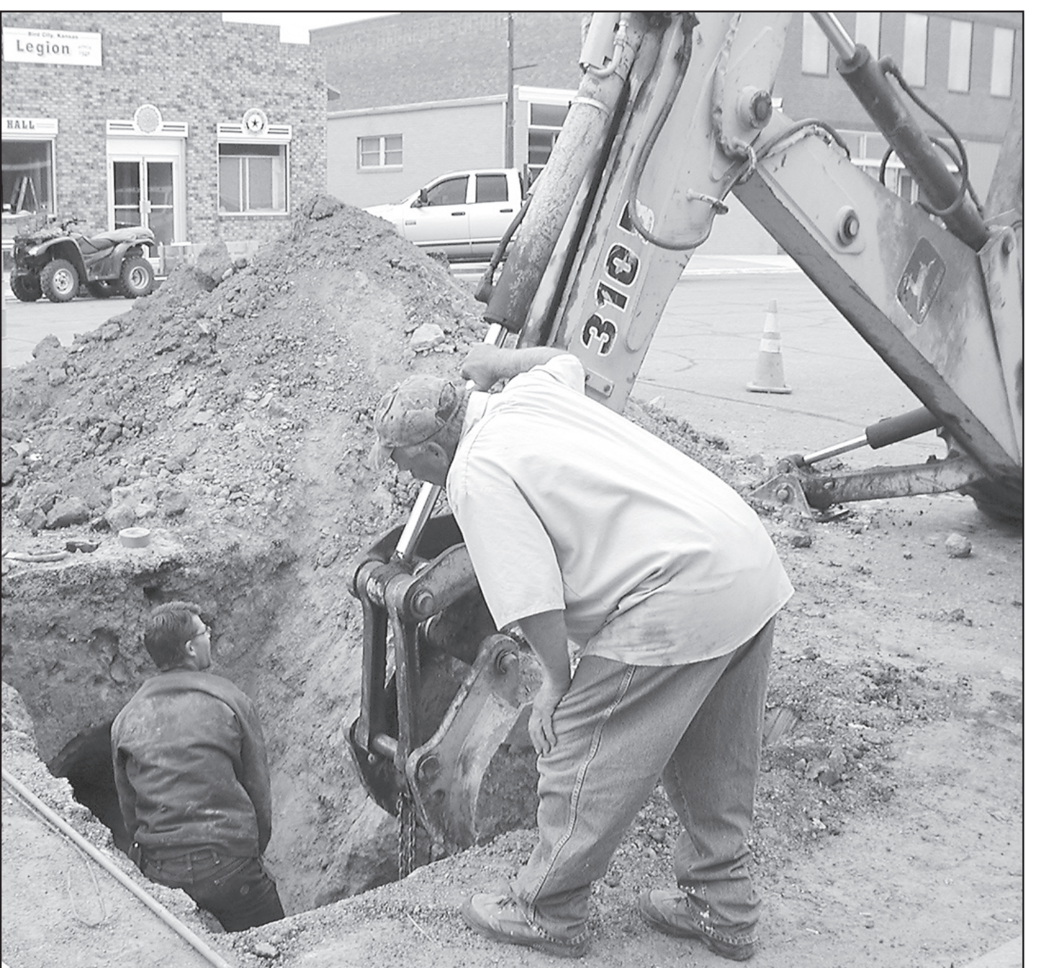
BRAD SCHNEIDER, Russell Jackson and Roy Shrader replacing the three-quarter inch water line with one-inch pipe. Times staff photo by Norma Martinez
